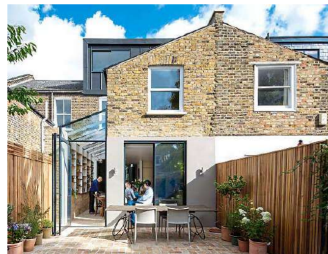
Transformation: An extension has opened up the ground floor
